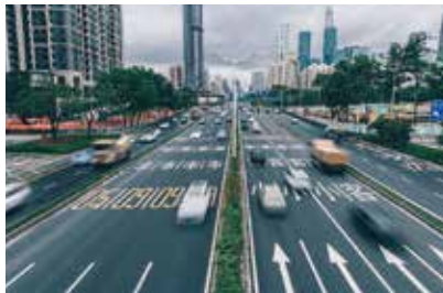
Intelligent Traffic & Safety Monitoring
