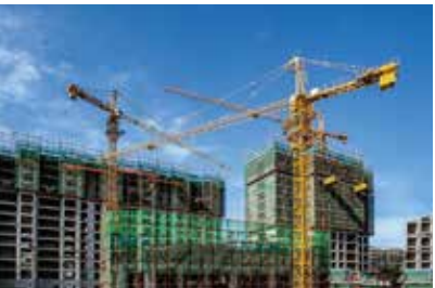
Construction Survey & Engineering Monitoring
