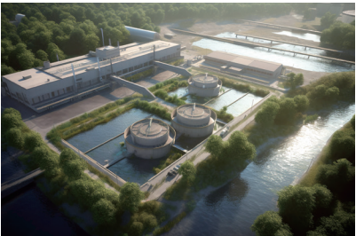
Water treatment industry
